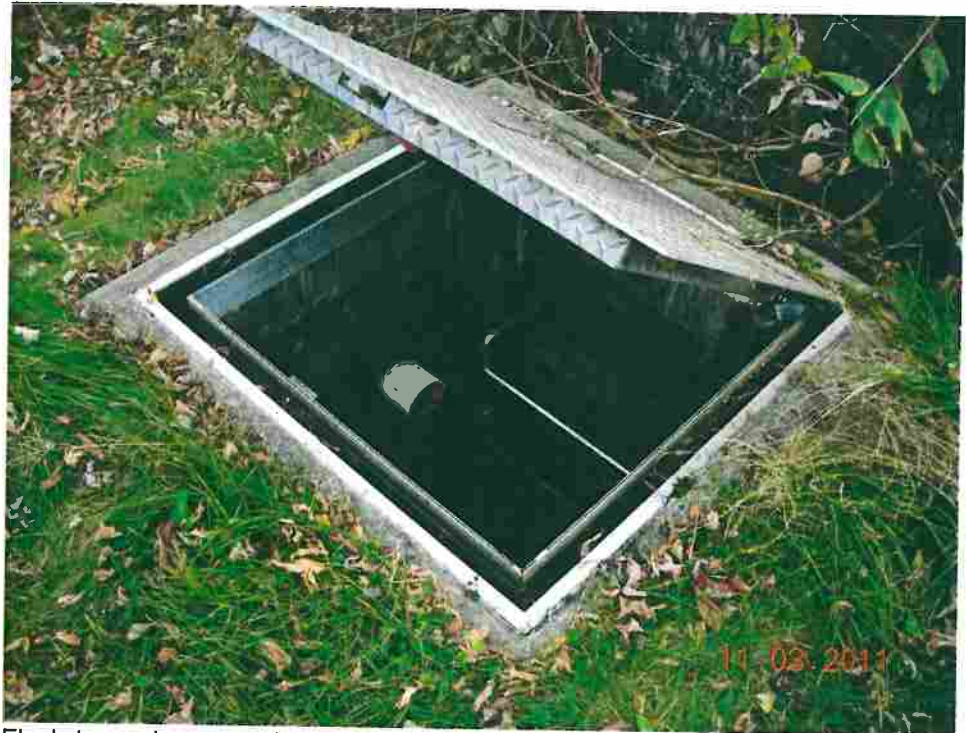
Flush to grade access hatch - tank is shown overflowing, wasting chlorinated "treated" water to Lake Champlain
