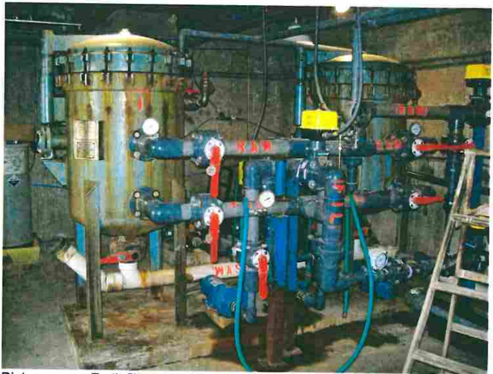
Diatomaceous Earth filter vessels, covered with rust and visible holes forming
