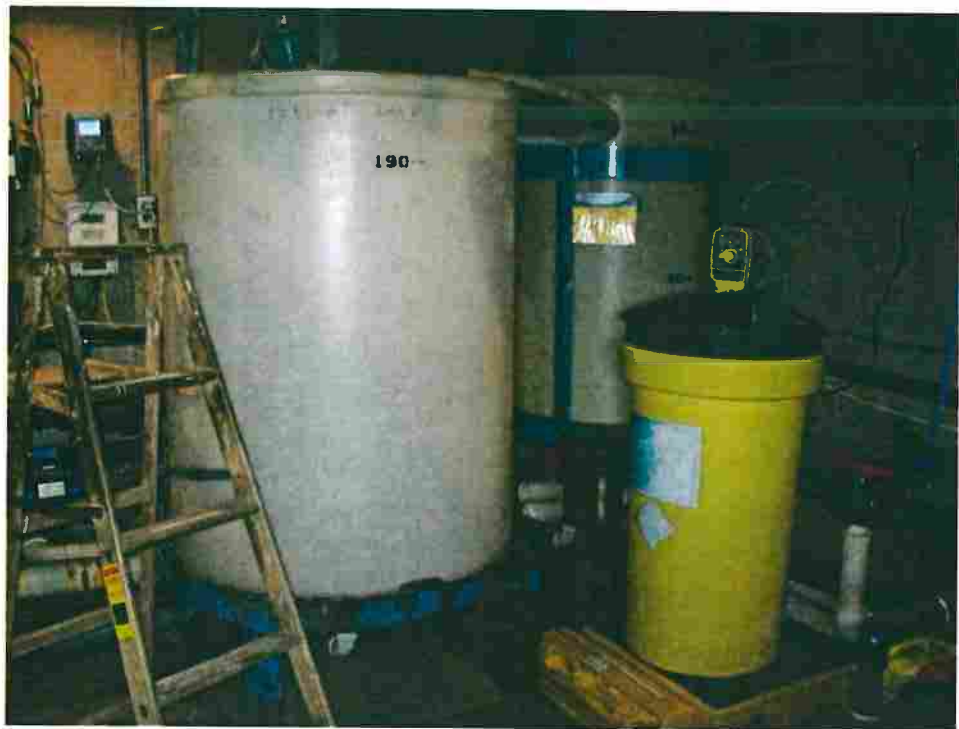
Unvented chlorine contact tank with single chemical feed pump
