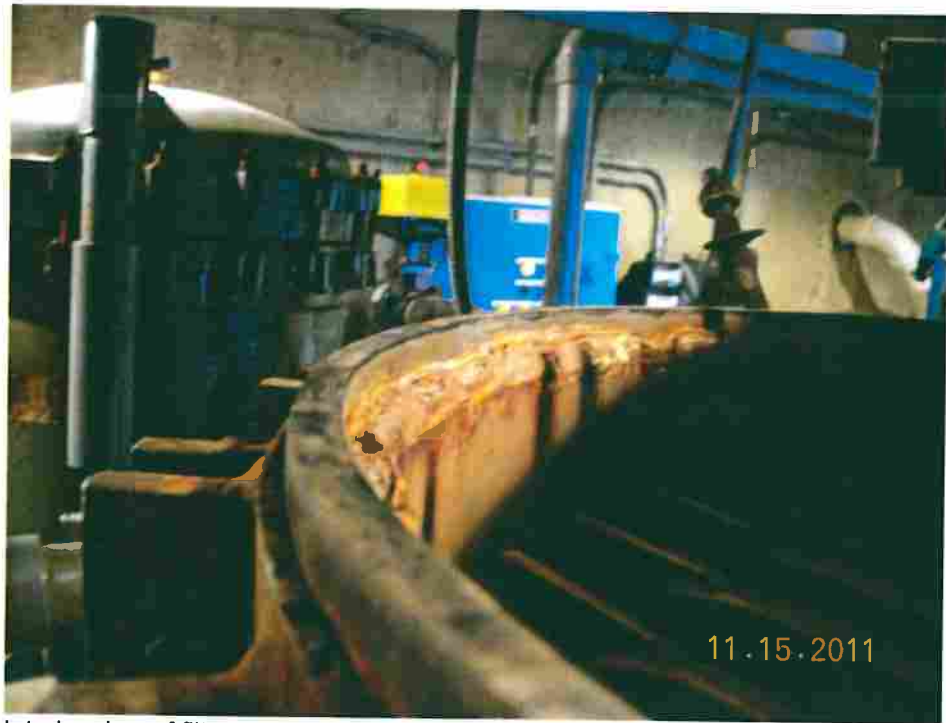
Interior view of filter currently taken out of service
