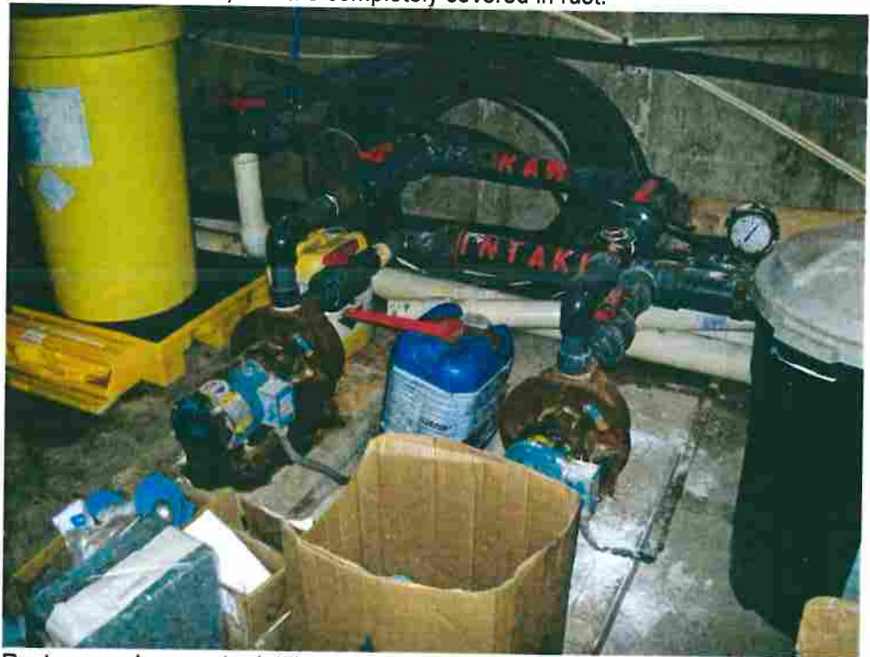
Rust covered raw water intake pumps
